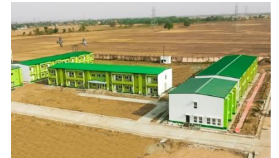
Light-gauge Steel Frames
