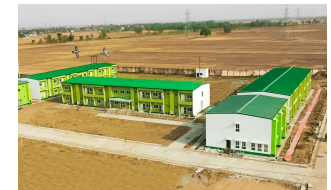
Light-gauge Steel Frames
